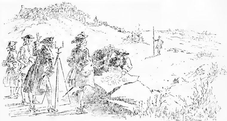
SURVEYORS LAYING OUT BALTIMORE
